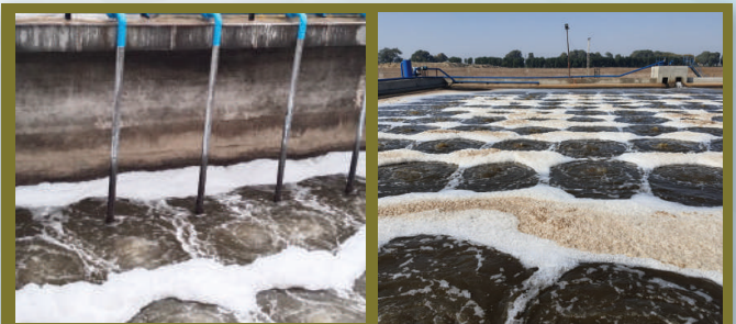
Typical UEE SBR System in operation
